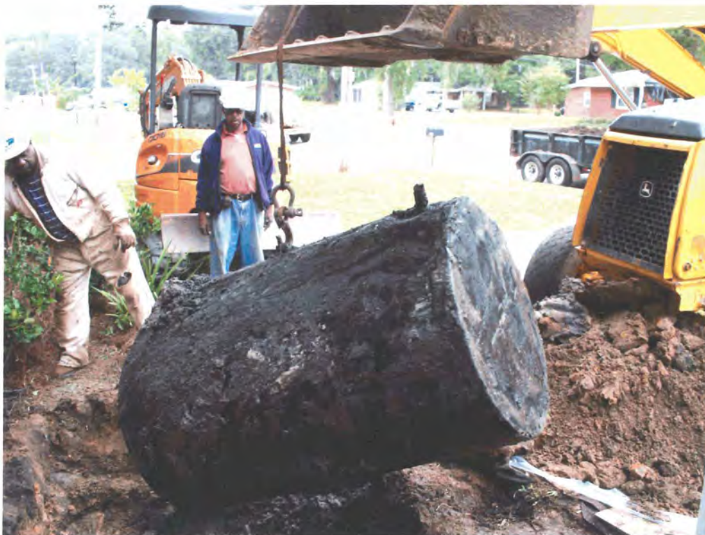
Picture 2: UST 444Elderberry-1 being removed from the excavation.
